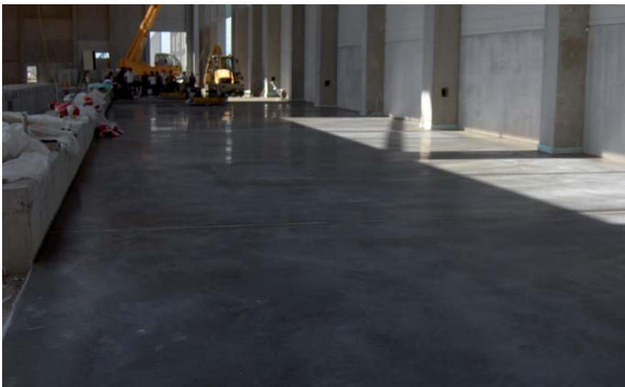
Figure 2: Completed floor slab.
