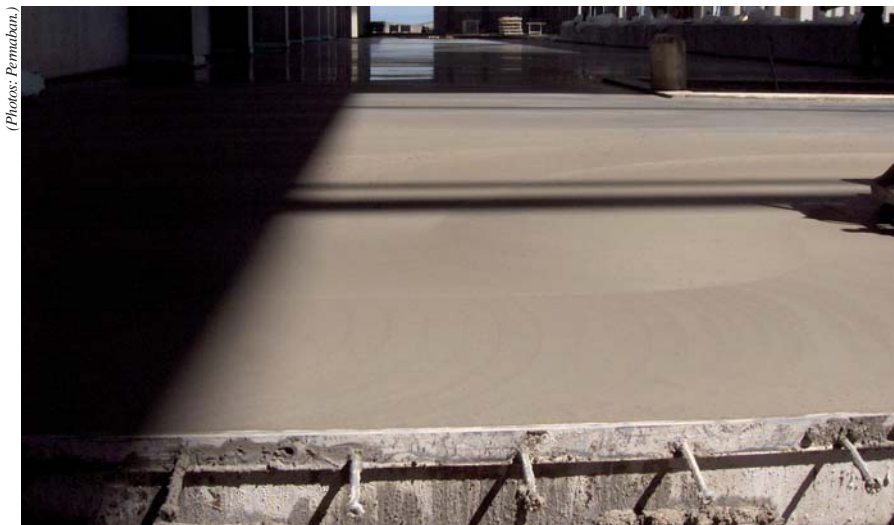
Figure 1: Recently power-trowelled floor.
