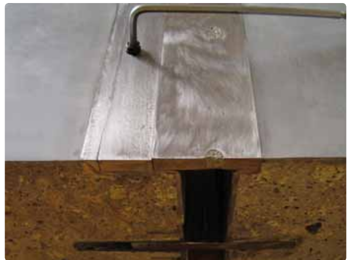
Figure 2 top left: Edge of post-tensioned slab adjacent to the dock levellers at Morrison's warehouse, Kettering showing the installed joint without the final wearing plate.
