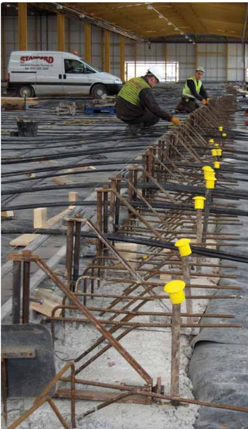
Figure 1: Joint close-up and general view of the AlphaFix joint levelling and post-tensioning cables at Morrison's warehouse, Kettering.
