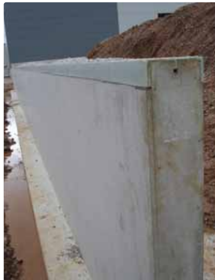
Figure 1 above: Precast dock leveller after four years in a busy distribution centre. Note the AlphaJoint approximately 1.5m away.
