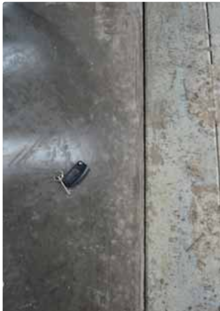
Figure 7 below: As Figure 5 after casting. The joint between floor and dock leveller has opened and is protected by Strip Joint.
