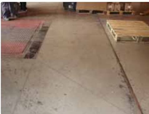
Figure 1 above: Precast dock leveller after four years in a busy distribution centre. Note the AlphaJoint approximately 1.5m away.
