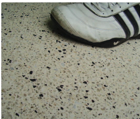
Figure 5: Finishing processes, such as diamond grinding and polishing, offer resilient and sustainable floors for almost any application.
