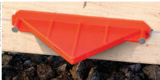
Figure 1: The Diamond Dowel sleeve is fixed to the timber formwork just prior to pouring the concrete.
