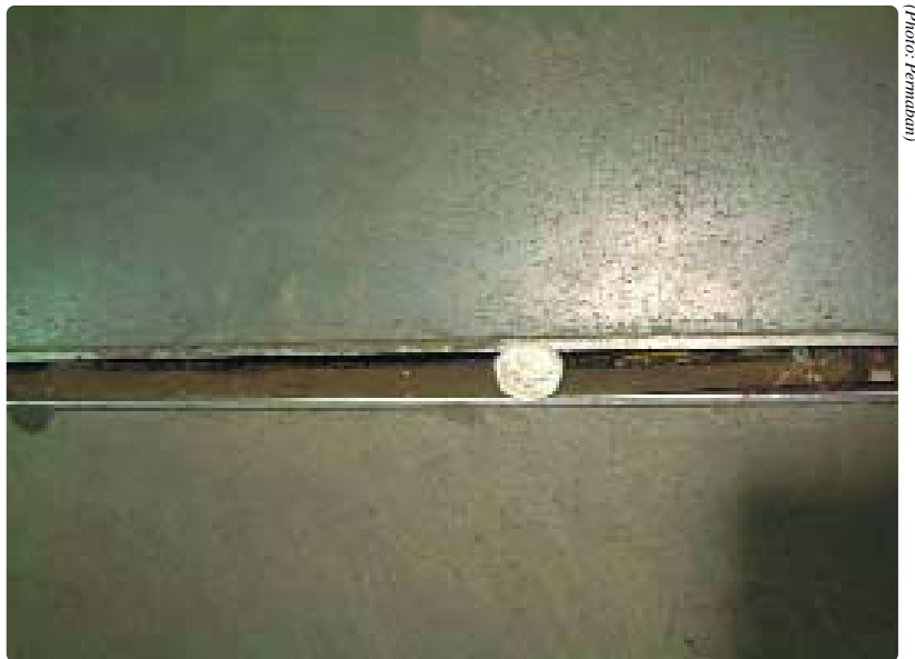
Figure 5: A formed joint on a ground-bearing slab showing a 25mm opening.
