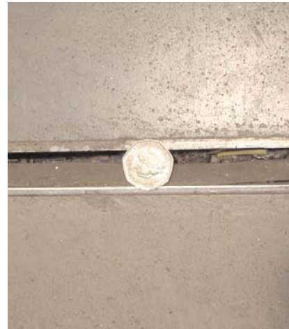
Figure 5: A 10mm section AlphaJoint in a busy transport warehouse. Note how the floor slab contractor has finished the concrete to the correct level and not buried the steel profiles.
