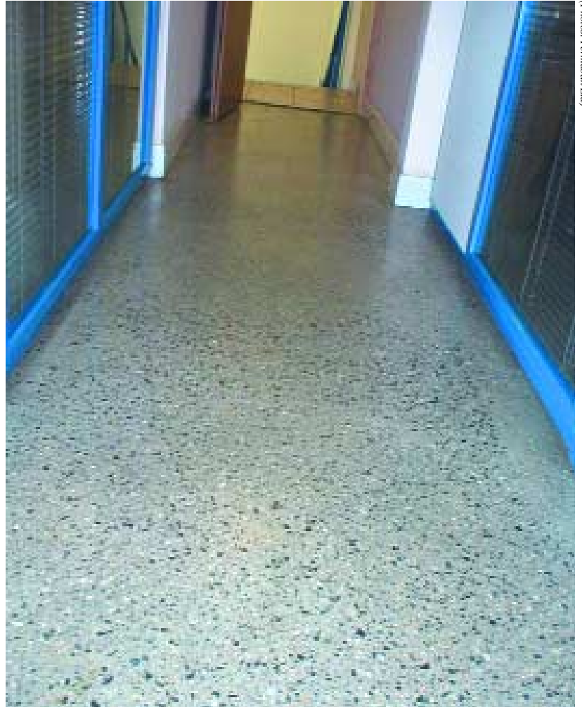
Figure 1: Diamond grinding greatly enhances the aesthetics of the finished floor.
