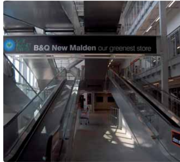
Figures 2 and 3 far left: Interior floor area in a new flagship DIY store. The floor has been cured with Aquacure.
