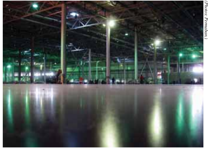
Figure 2: The completed first floor area at Southgate Industrial Park.
