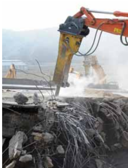
Figures 5 and 6: Secondary breaking of material. Hydraulic cutters and pulverisers break concrete and reinforcement bar in one step.
