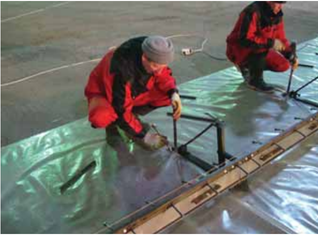
Figure 1: Installation of AlphaJoint GD8 at Southgate Industrial Park, near Moscow, Russia.
