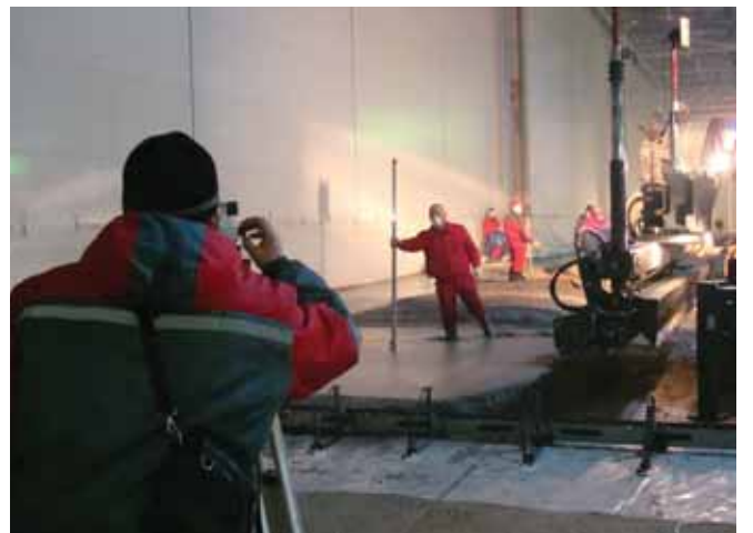
Figure 4: Check and recheck of the floor levels.
