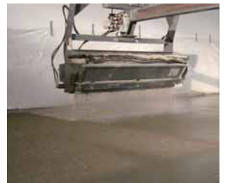
Figure 6: Application of DryShake Floor Hardener.
