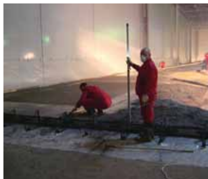
Figure 5: Checking the level of the AlphaJoint.
