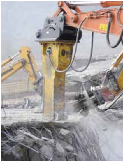
Figures 5 and 6: Secondary breaking of material. Hydraulic cutters and pulverisers break concrete and reinforcement bar in one step.
